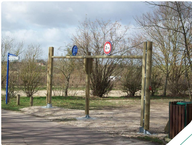
Height restriction gantry with central locking for - Portugal
