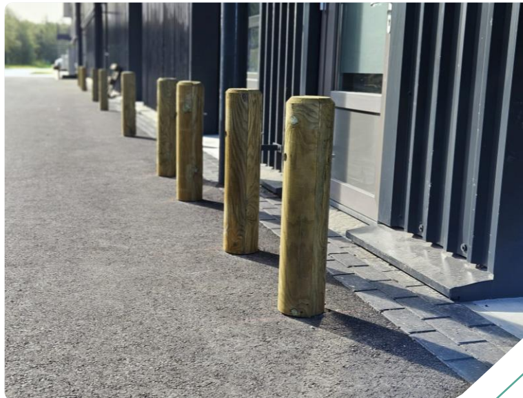
RICANTO bollards - Netherlands
