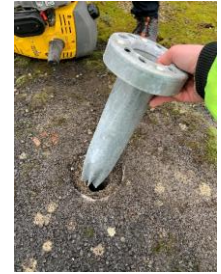
Step 4: Insert the anchor piles into the ground
