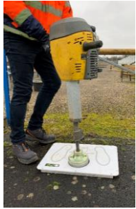
Stage 1: demarcation of the insertion area by impression or decoring
