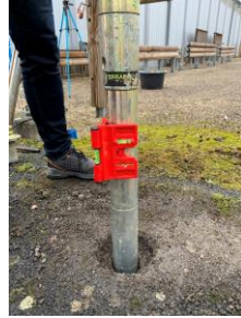
Stage 2: drive down the hole in the ground - check axial alignment
