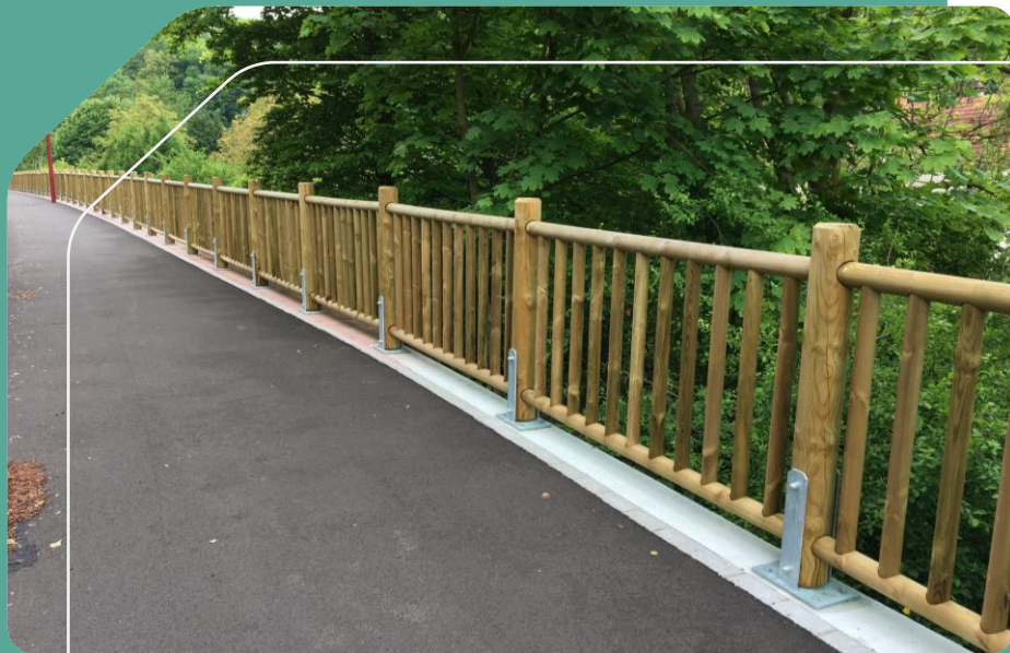
Example of hot-dip galvanized anchoring
