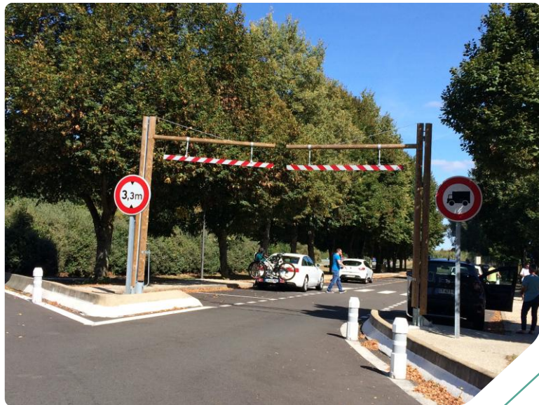
Gantry - COFIROUTE motorway service areas (France)
