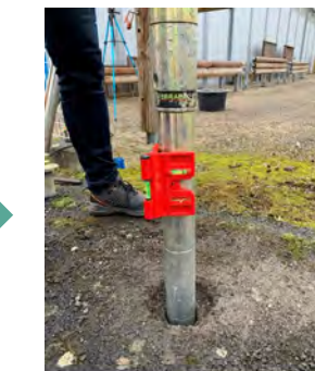
Stage 2: drive down the hole in the ground - check axial alignment
