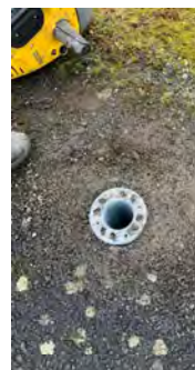
Stage 5: intermediate check of the straightness of the pile in the ground
