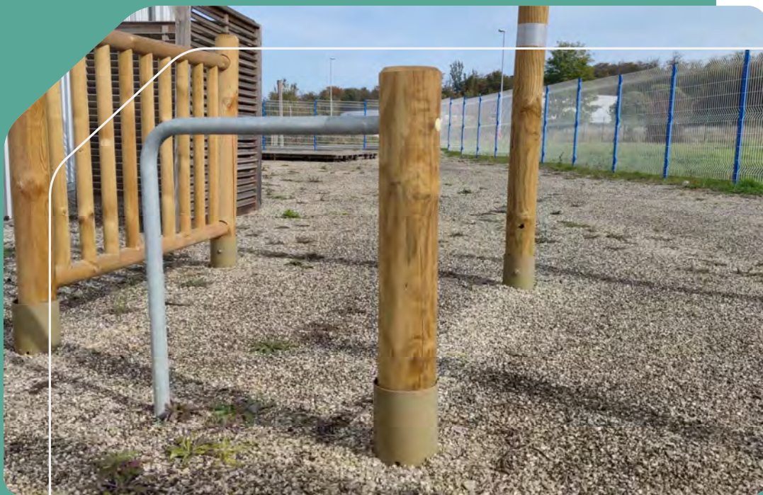
Powder-coated sleeve RAL 7008
