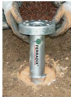
CITY anchoring piles Addition of 20% of concrete
