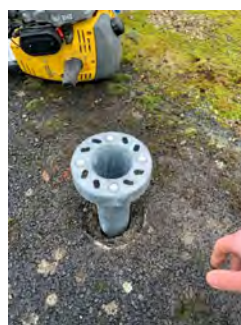
Stage 5: intermediate check of the straightness of the pile in the ground
