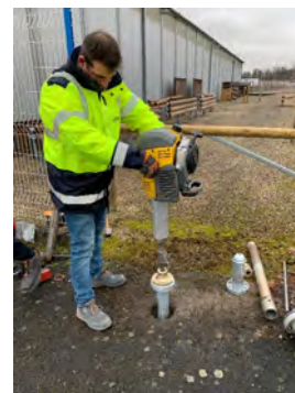
Stage 3: drive in the anchor piles using a pneumatic hammer and dedicated installation tool.
