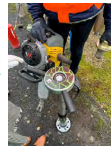
Step 4: Insert the anchor piles into the ground
