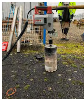
Stage 1: demarcation of the insertion area by impression or decoring
